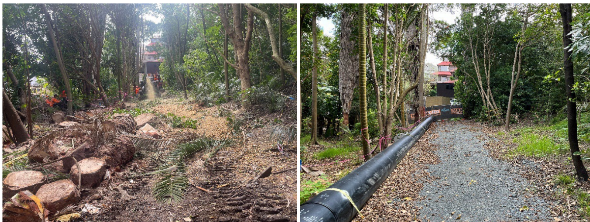
Figure 3: Vegetation clearance (Left) and temporary accessway and WW diversion (Right).
