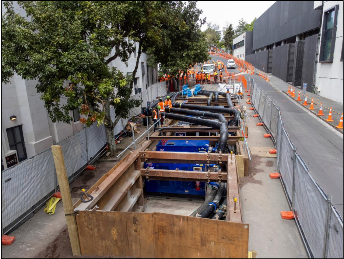
Figure 7: Diversion pumps installed on St Georges Bay Road.
