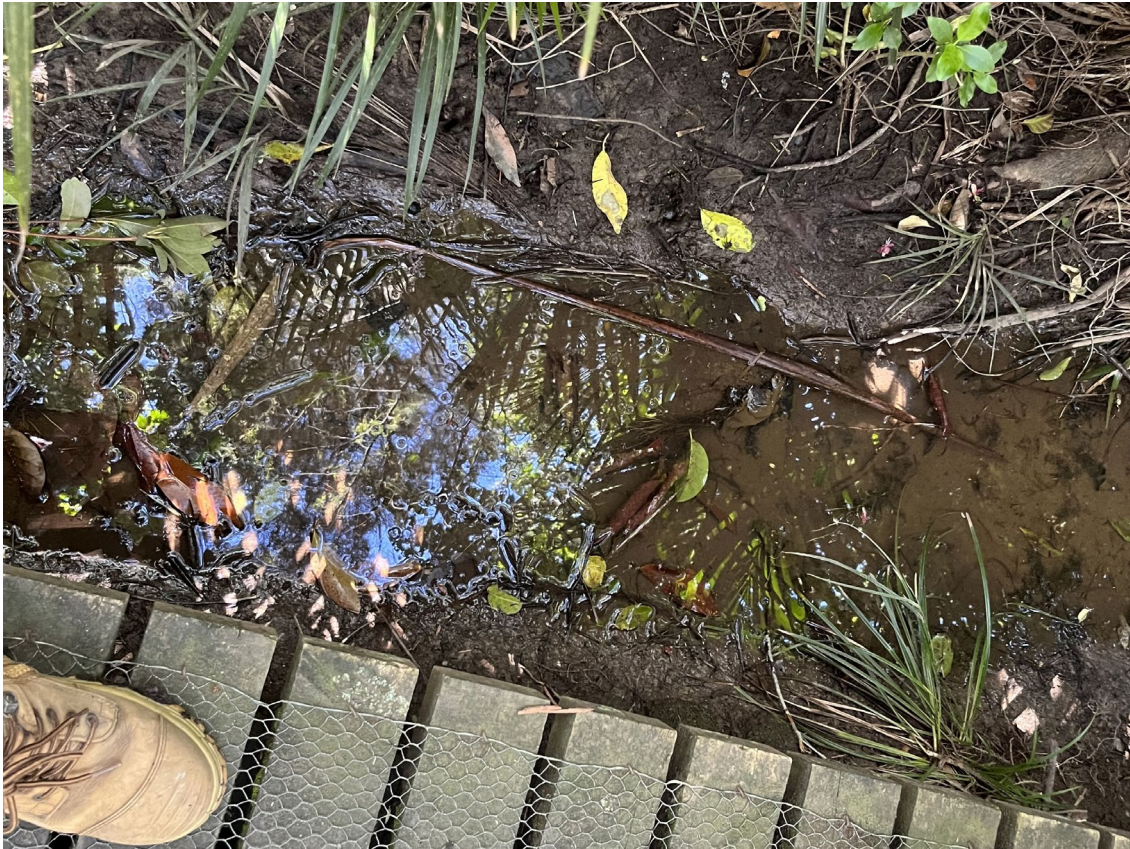
Figure 3: Evidence of pooling.
